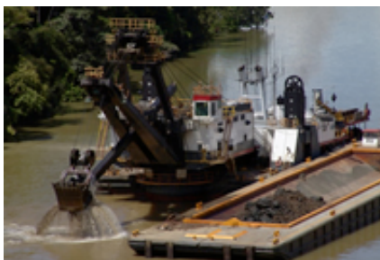
The Army Corps of Engineers proposes dredging dioxin-contaminated sediments from the Upper Saginaw River and disposing these sediments on a floodplain in Zilwaukee, Michigan. Above, a navigational river dredging operation. Photo: Shutterstock.
